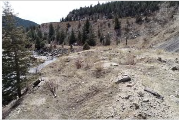
Exhibit 10. Existing I-70 Roadway Embankment
